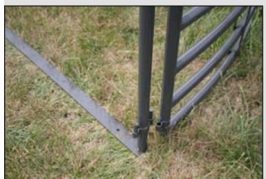
Retrieve second curved panel and attach to secondary bow at end of first curved panel.
